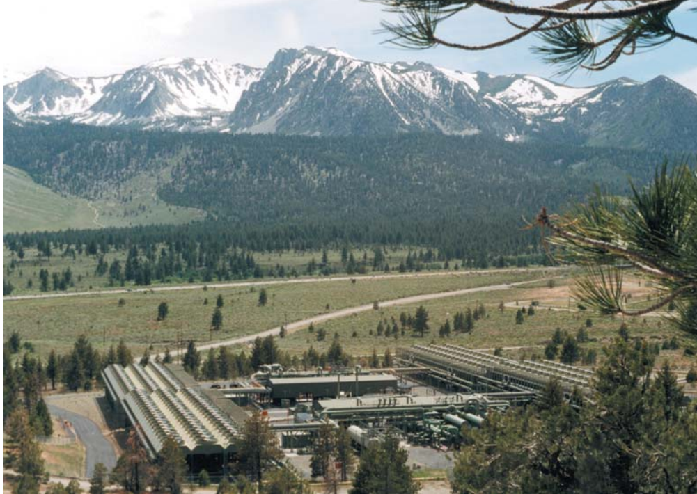
The Mammoth Lakes Power Plant is located in a picturesque area of northern California. Binary-cycle geothermal power plants release no carbon dioxide or water vapor plumes and blend into the environment.
