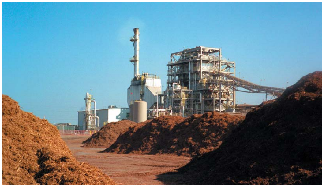
Andrew Carlin, Tracy Operators, NREL PIX 06665
