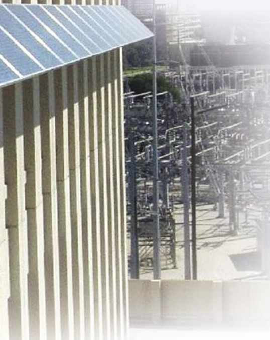
This 7-kW PV awning generates electricity and also provides shading that offsets part of the air-conditioning load. (credit: University of Texas Health Science Center at Houston)
